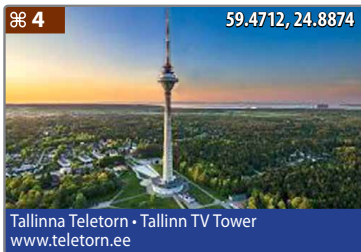
4 59.4712, 24.8874 Tallinna Teletorn • Tallinn TV Tower www.teletorn.ee
